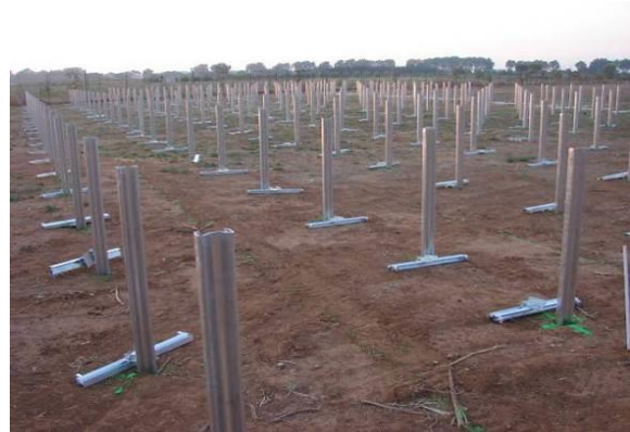
Aspect des supports
